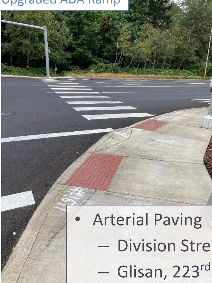
Upgraded ADA Ramp
