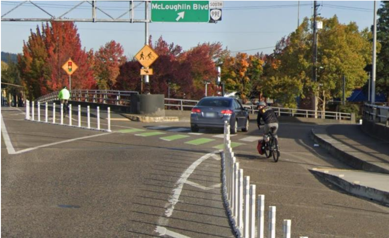
Before 2024 Paving Project:
