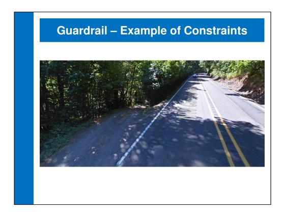
This a picture of just one location on Cornelius Pass where the design team will have a challenge with guardrail installation. This location is a steep driveway where a break in the guardrail is needed and where it may be challenging to provide acceptable end treatments for the guardrail.
