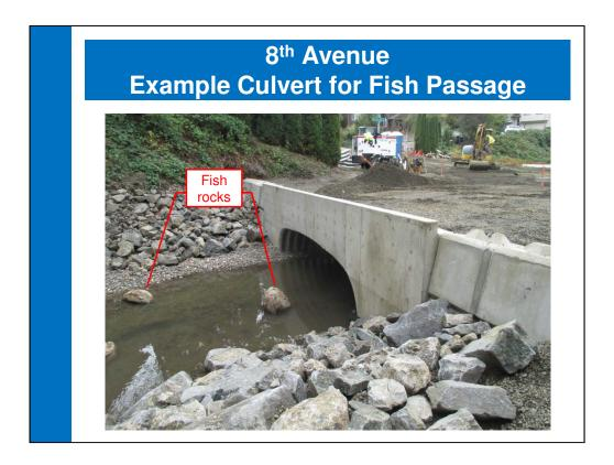
This picture is an example of what the stream and culvert could look like to accommodate fish passage, however, we will likely end up with a box culvert instead of the steel arch shown.
