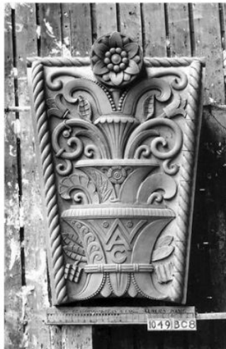
Architectural decoration (Gladding McBean, 1930) for Washington Athletic Club building
