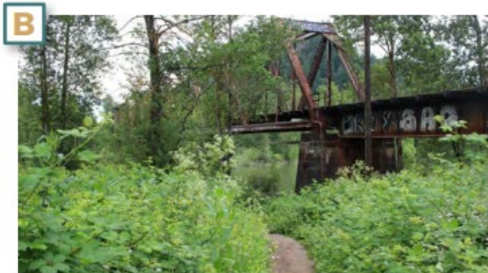
Current access to the site under the railroad trestle to the site, connecting to the future bike hub, visitor's center and Downtown
