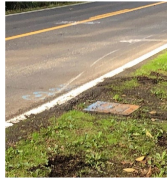
Figure 10. Existing drain in SE Lusted Road right-of-way
