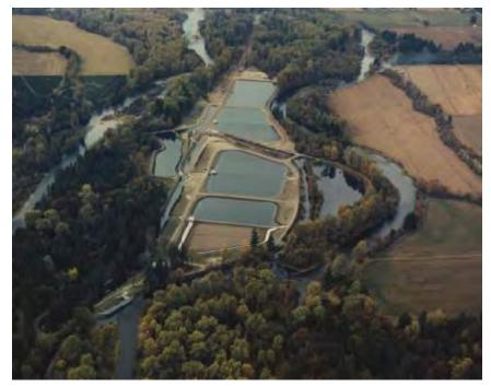
Slow sand filters can be differentiated from standard granular media filters by the following characteristics:
