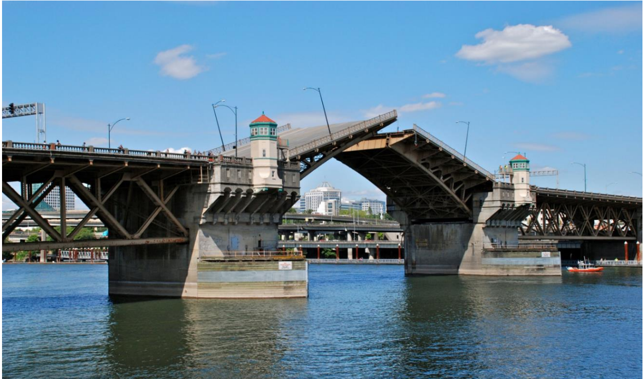
Figure 1. Burnside Bridge Main River Span Bridge over the Willamette River, Portland, Oregon
