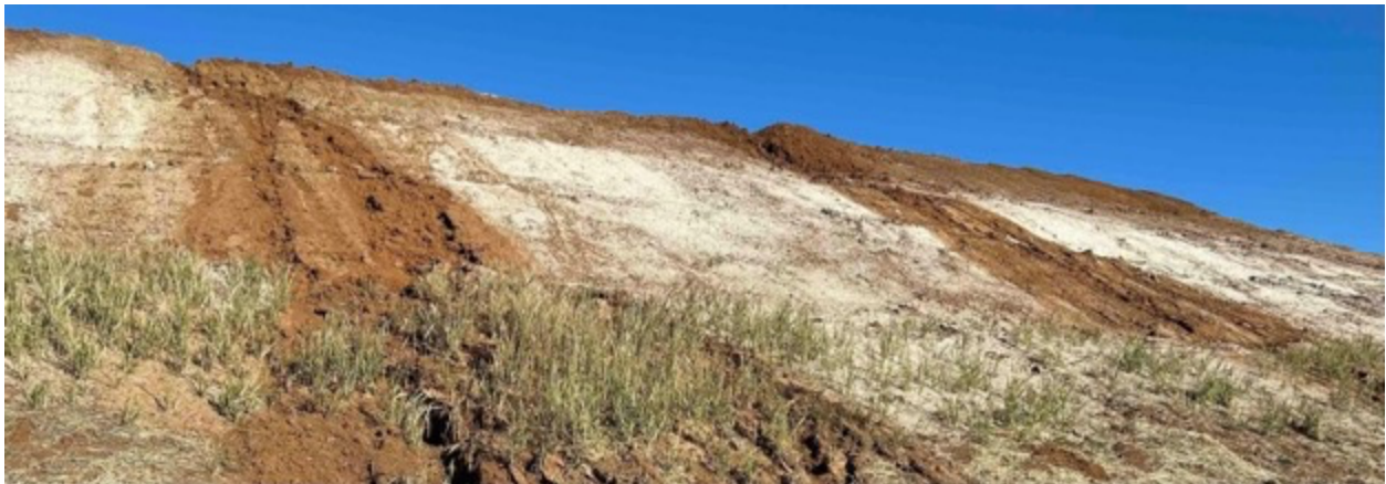
Figure 3. Example of erosion occurring on stockpiled soil at PWB's construction site.
