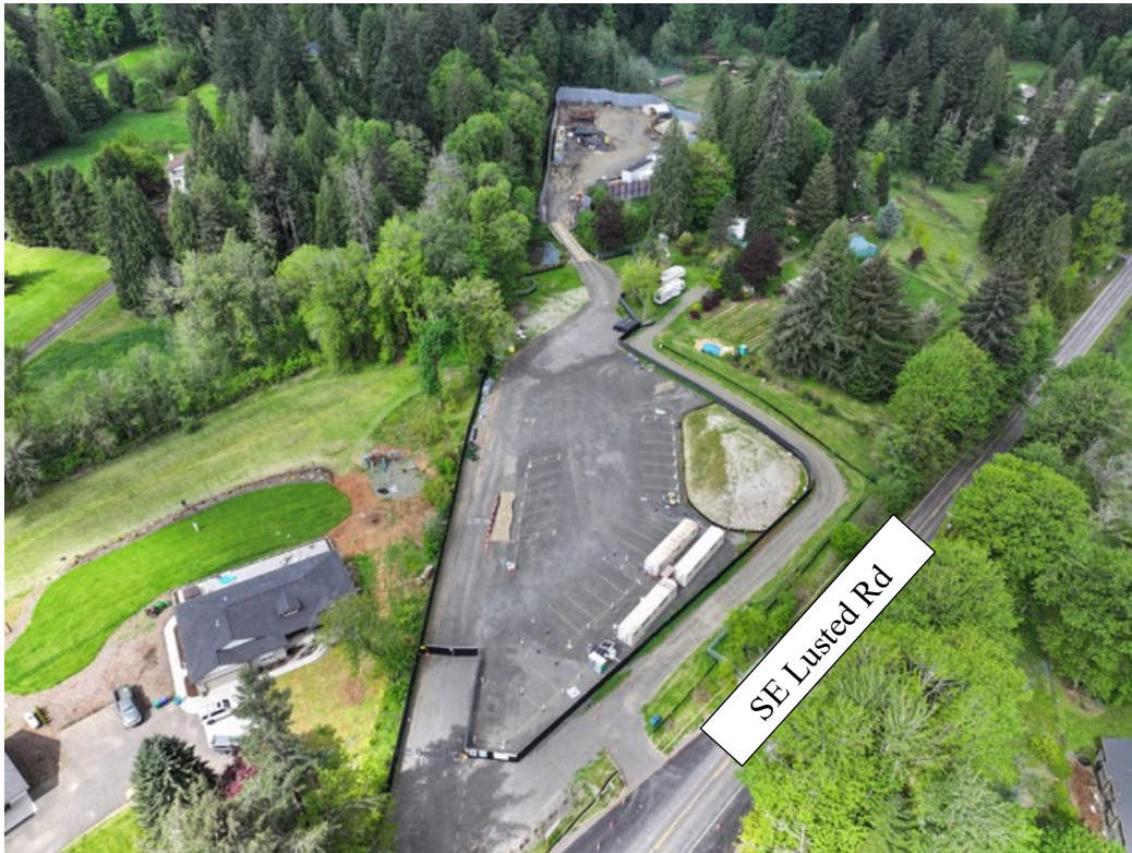
Figure 2. Raw water portal site looking west from SE Lusted Rd, May 2025.
