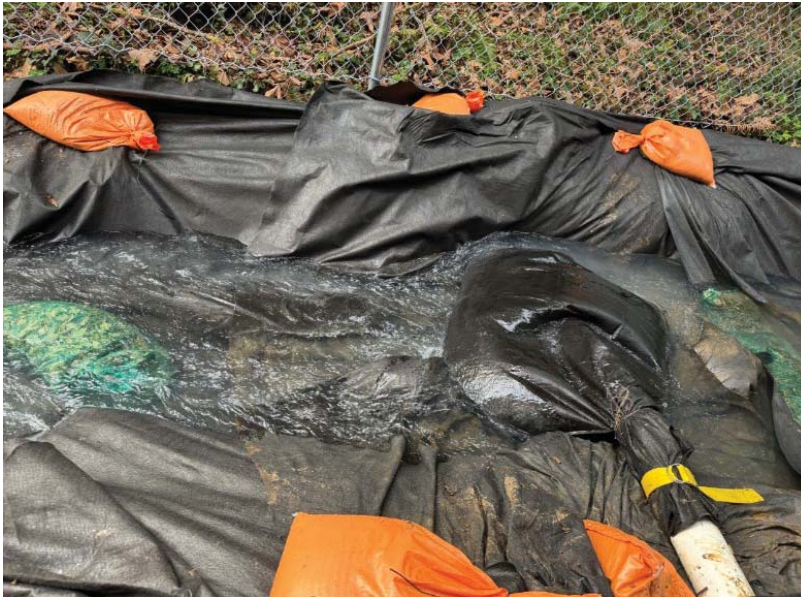
Photo 12: Taken March 24, 2025, showing clear water from the sump pump and 6" HDPE line filtered through sediment filter bags prior to entering the catch basin and discharging to the culvert across SE Lusted Rd
