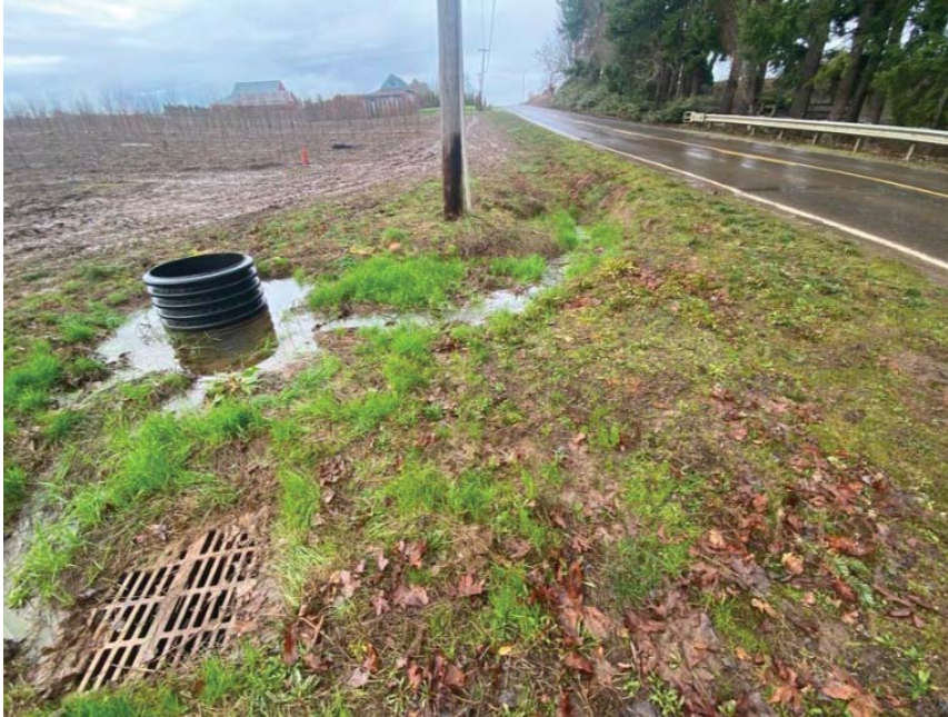
Photo 4: Taken February 9, 2023 showing excess drainage around the pre-existing collection system and unprotected catch basin prior to conducting work
