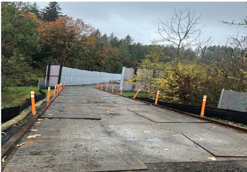
Photo 15: View of hardened road structure with sediment fence and straw wattles on each side.
