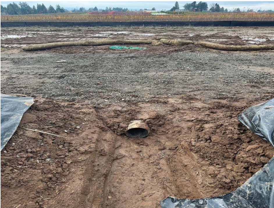
Photo 17: Taken November 26, 2024, showing installation of pipe to help convey water off the Schoepper property as pre-construction would have normally drained.
