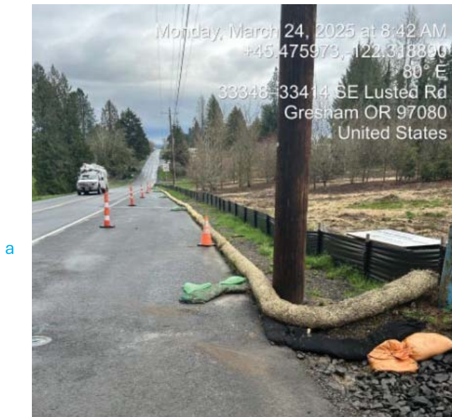
Photo 10: Taken March 24, 2025, after the rain event on March 21, 2025. In contrast to Photo 8, this photo shows no water running down the shoulder of SE Lusted Road. As noted in Photo 8, between Photo 8 and this photo, a berm was built forcing the water to a small well with a pump that discharges water back to the grated catch basin after passing through filter bag.
