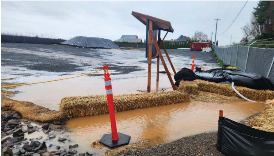
Uncontrolled water runoff into Beaver Creek from the PWB Lusted site. March 21 2025
