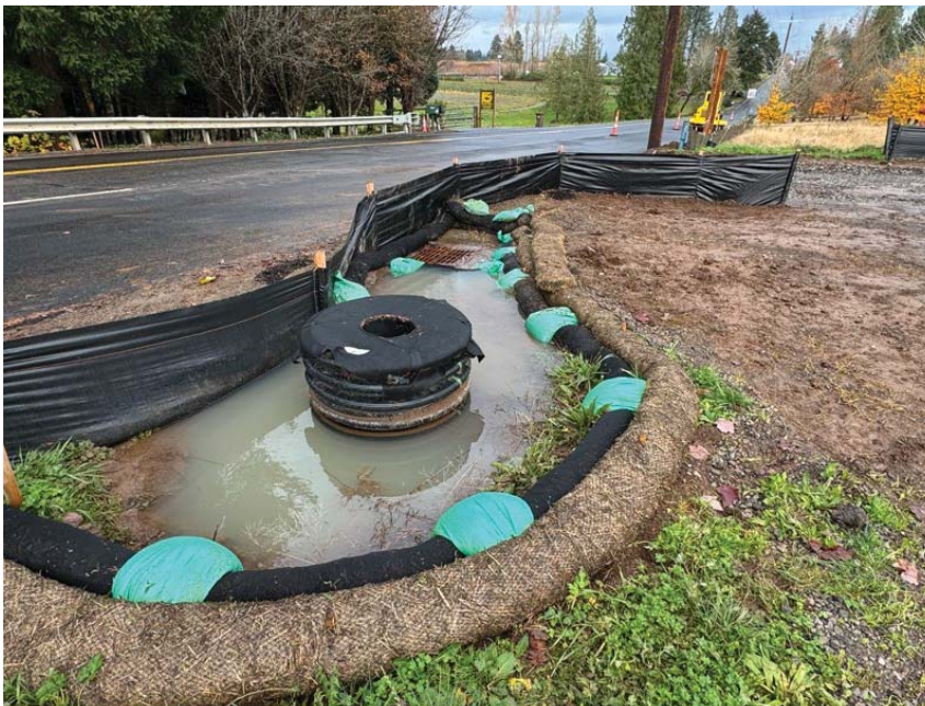
Photo 5: Taken November 13, 2024, showing construction stormwater management improvements surrounding the pre-existing vertical HDPE pipe in the foreground and grated catch basin behind.
