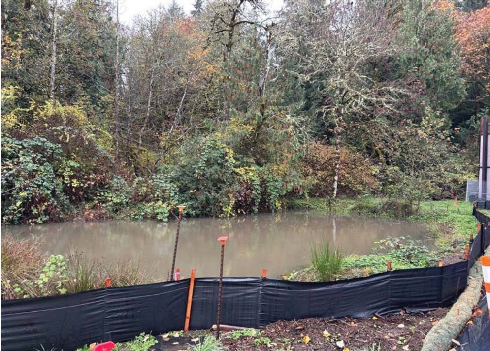
Photo 14: Silt/Sediment Fence installed at delineated wetland boundary – Pond side of Hardened Road
