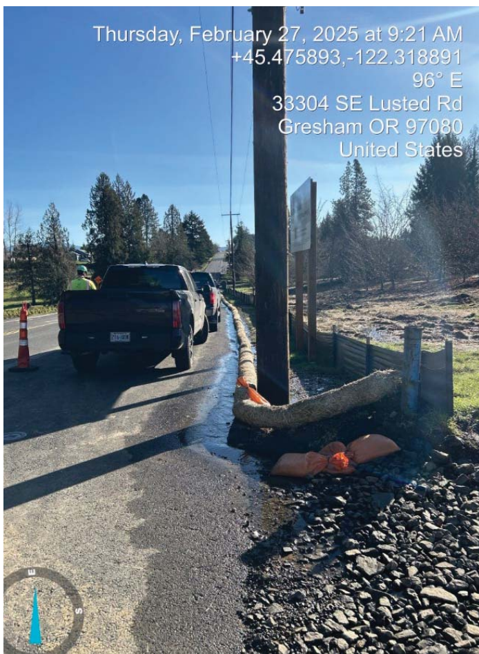
Photo 8: Taken February 27, 2025 shows water that was running under the FWI gravel pad and down the shoulder of SE Lusted Road. Since this picture was taken, a berm was built forcing the water to a small well with a pump that discharges water back to the grated catch basin.
