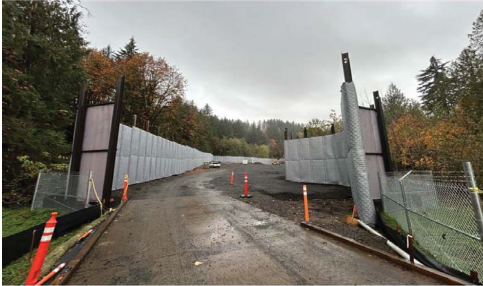
Photo 16: View of west end of hardened road with black sediment fencing below road protecting wetlands on each side from sediment/erosion. The taller grey fabric walls in background are sound wall material for noise mitigation during construction.
