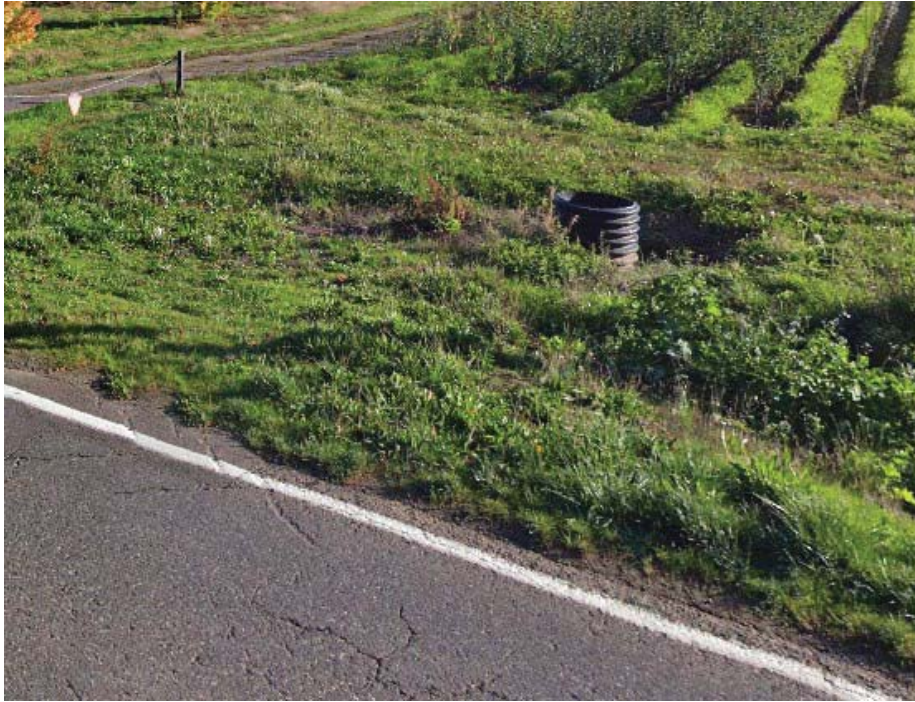
Photo 1: Image from Google StreetView from October, 2023 (Pre-Construction) showing vertical HDPE pipe installed by property owner
