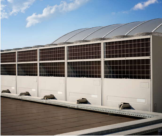
Figure 24: (Left) Air Cooled Variable Refrigerant Flow Condensing Units (Right) Package Air Cooled Rooftop Unit.
