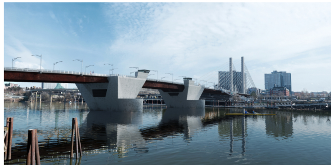
Conceptual rendering of the Preferred Alternative, the Replacement Long-Span Bridge. Example image showing a cable-supported bridge type option. A tied-arch bridge type option is also under consideration.
