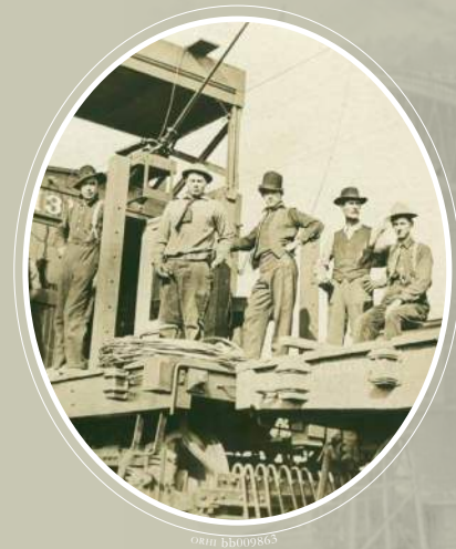
Construction began in January of 1925. Crews worked feverishly to meet the contracted schedule, which stated the new Sellwood Bridge was to be completed in just 250 working days, before the end of the year.
