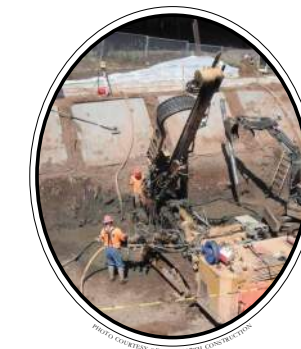
Workers drilling holes for ground anchors on concrete blocks.
