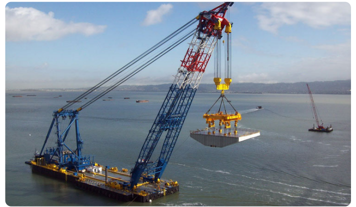
Our team's experience also includes AB's design and construction of the "Left Coast Lifter" on the San Francisco-Oakland Bay Bridge SAS project. AB provided engineering for the heavy lift, structural steel erection, and falsework scopes.
