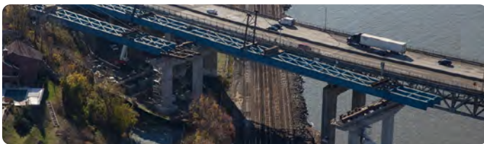
Traylor and AB supported engineering for over 40 marine cranes, four tower cranes, multiple cranes on work bridges, and land-based cranes. The team also designed temporary works to launch girders over Metro-North Rail to minimize impacts to commuters.
