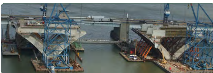
AB also provided in-house engineering for the falsework, shoring, and heavy lift of the bascule leaves on the Woodrow Wilson Bridge.
