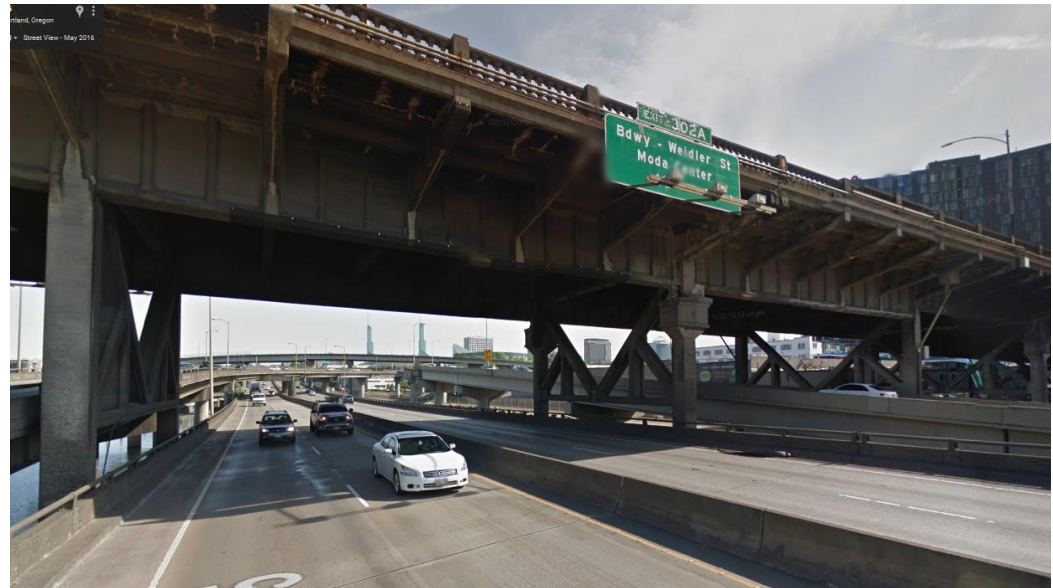
Photos of sections of bridge next to I-5
