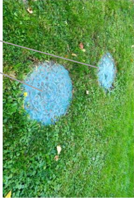
Septic Tank Manhole Cover
