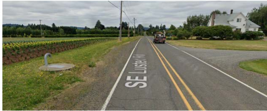
Figure 14. Example of Existing Air Vent and Access Vault (left) within Lusted Road ROW
