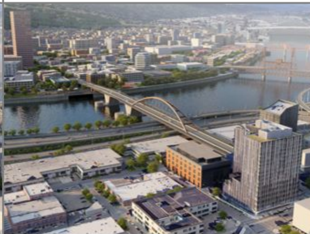
Braced basket-handle arch
