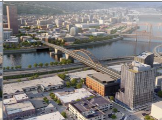
Braced vertical arch
