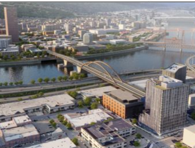
Unbraced through arch
