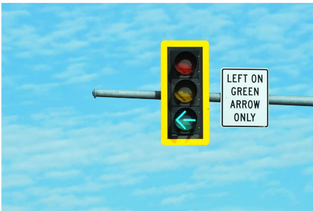
Protected or protected/permissive left turn phasing
