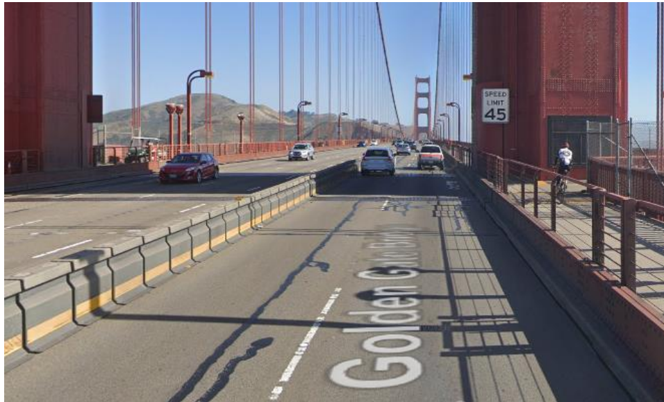
Figure 18. Reversible Lane Movable Barrier Example
