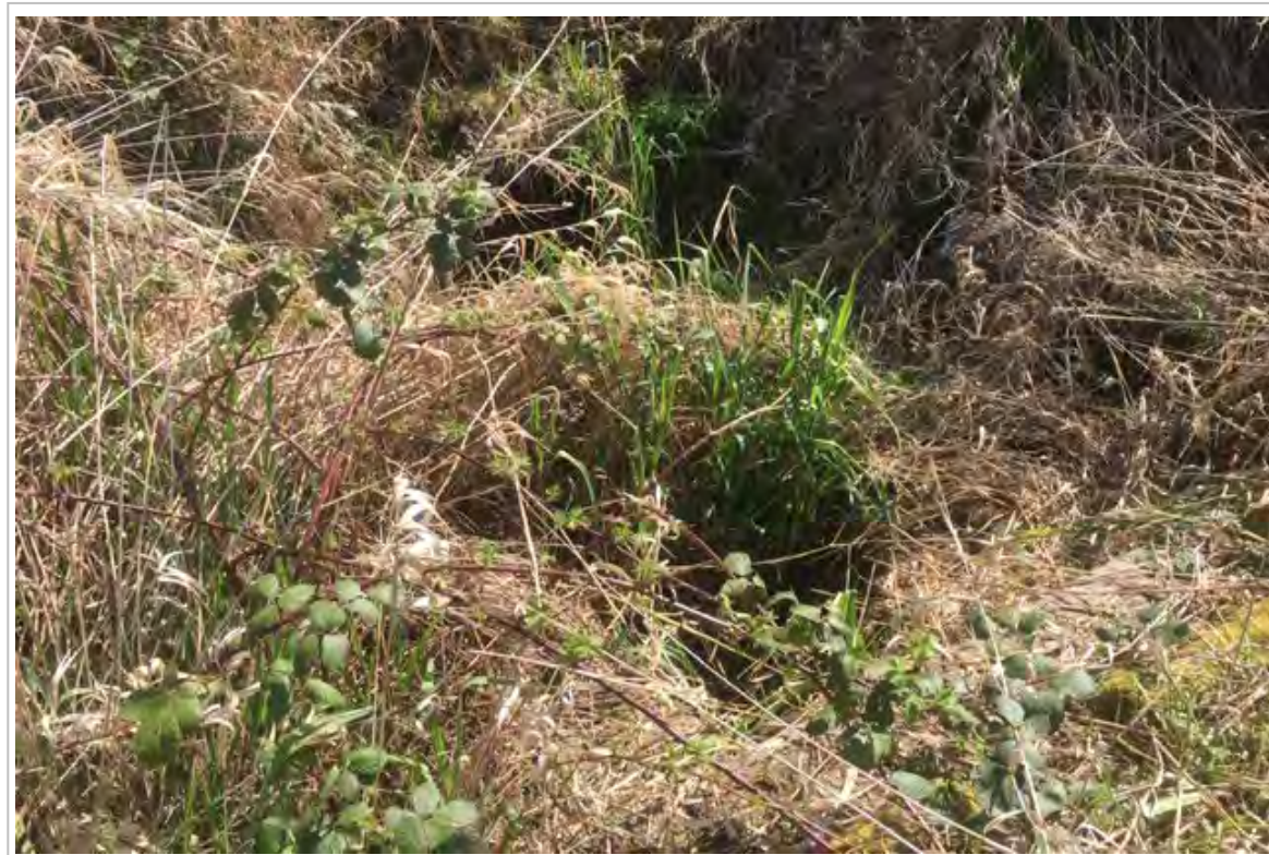
Photopoint 2: Culvert discharging from under Dodge Park Boulevard flows briefly at the surface before entering another culvert system. The break is to allow water from along the embankment to drain into the daylighted area and drain from the area.
