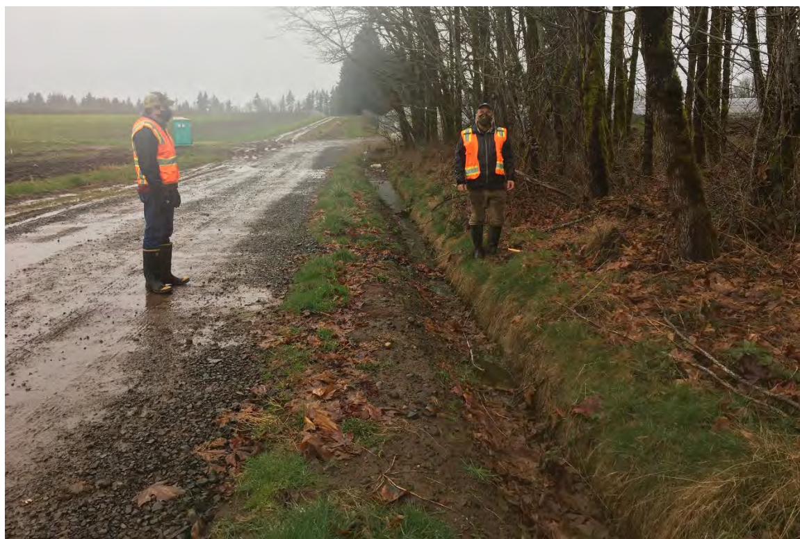
Photopoint 16: Southern end of ditch. Water flows in from upslope and sheet flow from adjacent farm access road.
