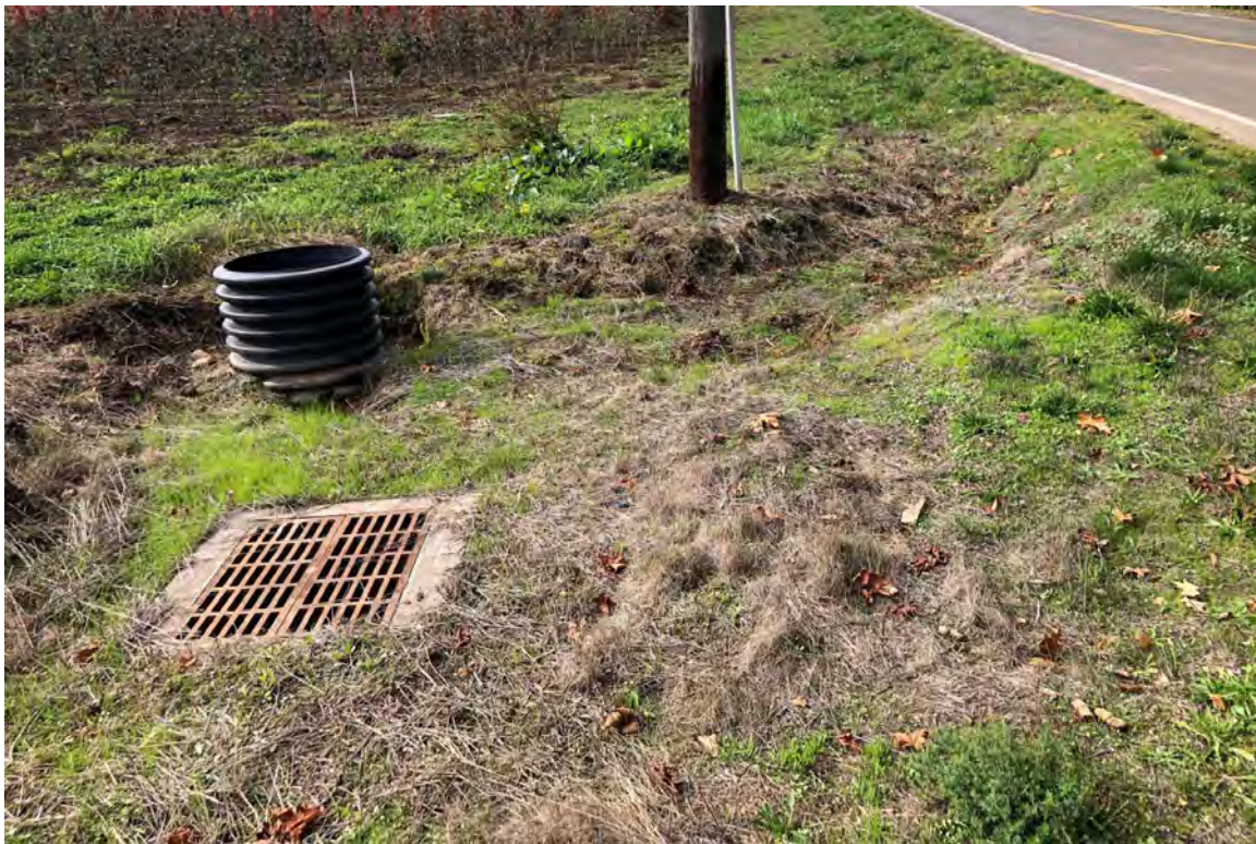
Photopoint 20: Plot 16 was taken in the low spot next to the stand pipe and area drain. Roadside ditch that drains into a small basin. Water is collected into the area drain and exported under Lusted Road to Beaver Creek.
