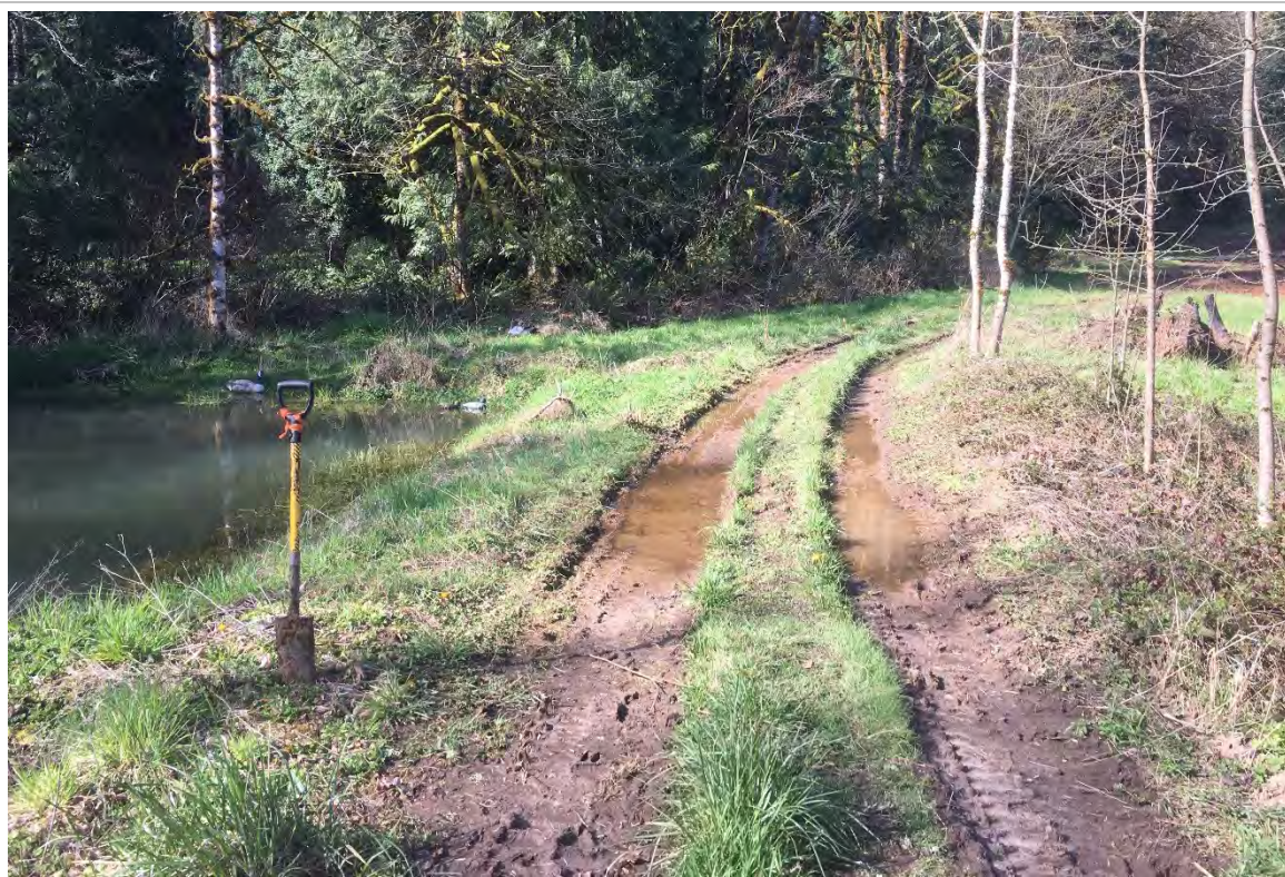
Photopoint 7: Looking southwest at a farm access road that passes between the two ponds (Waters 2 and 3 on Figure 5c). A concrete culvert conveys water from left to right under the road.
