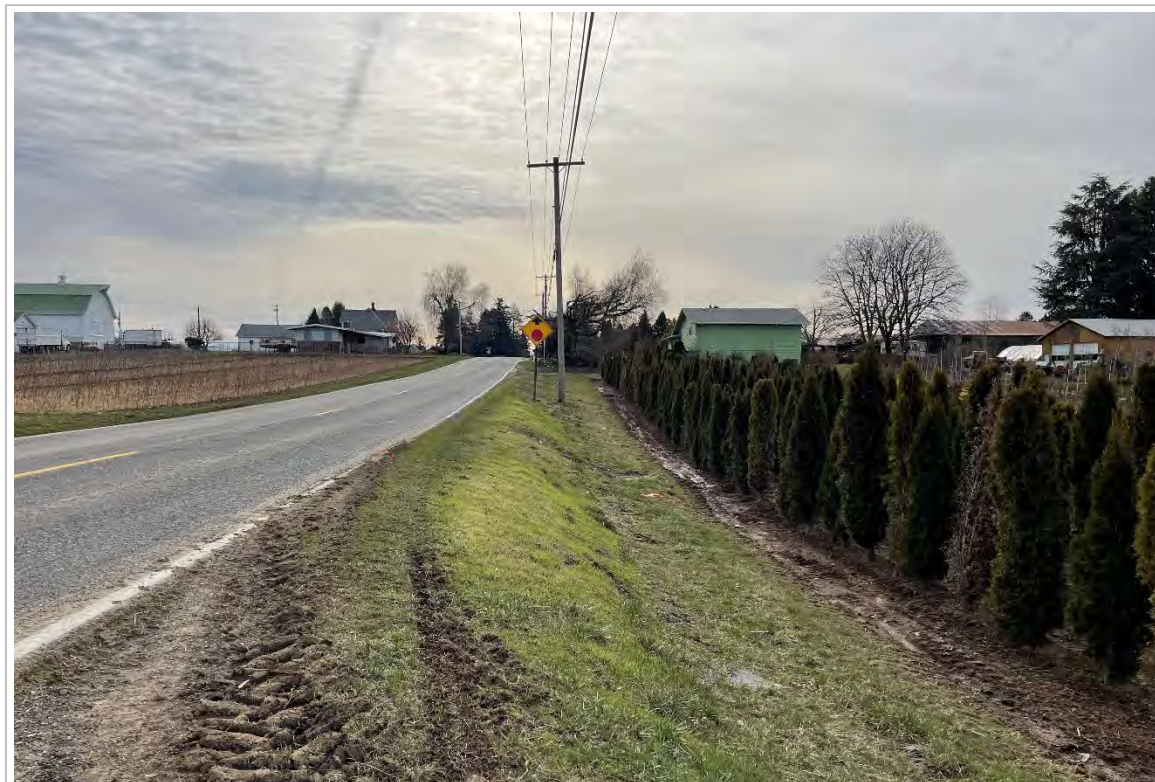
Photopoint 18: Opposite side of Altman Drive from Photopoint 17. Water from ditch above does not daylight, but is captured in a drainage system under the property west of Altman Drive.
