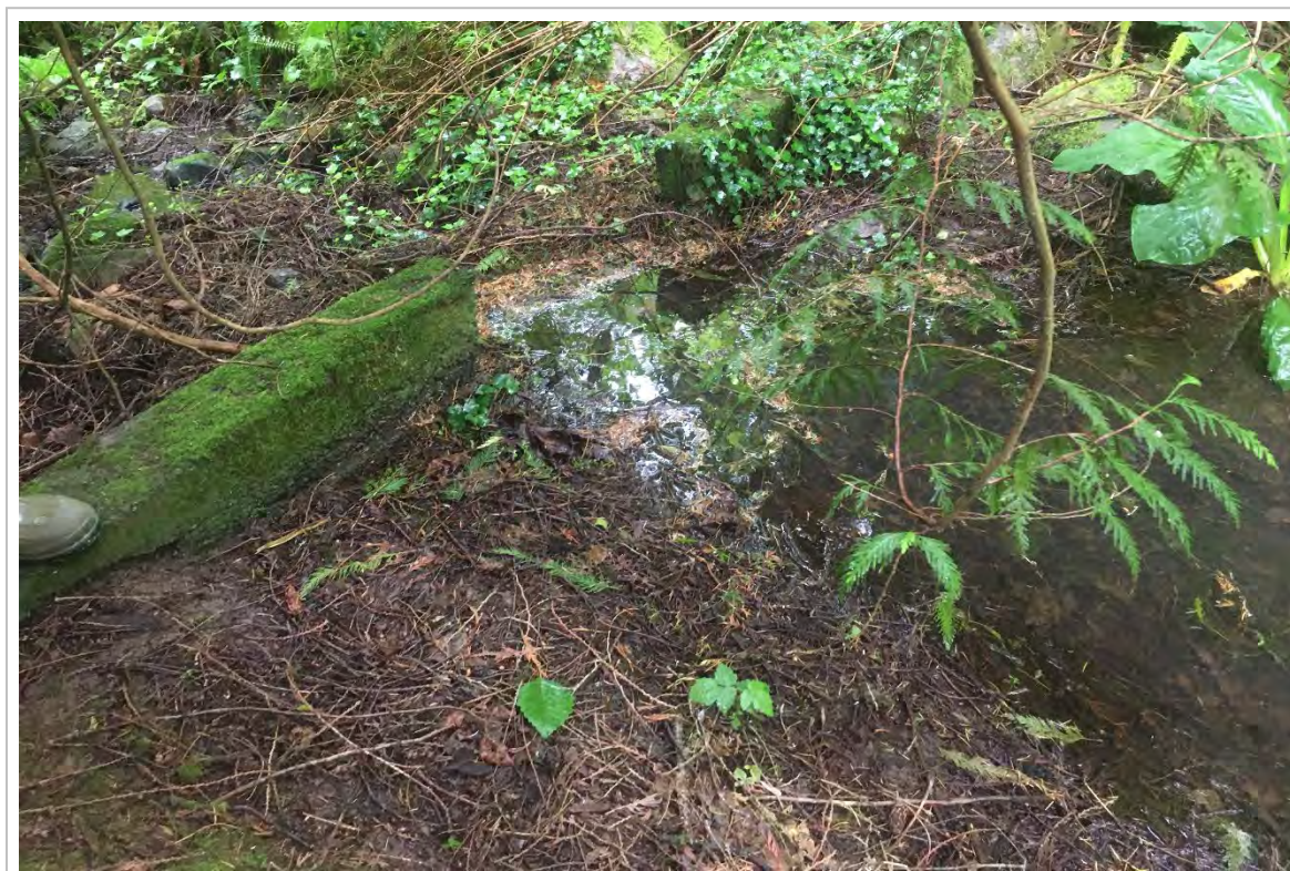
Photopoint 12: Old water control structure on Water 3, downstream of ponds.
