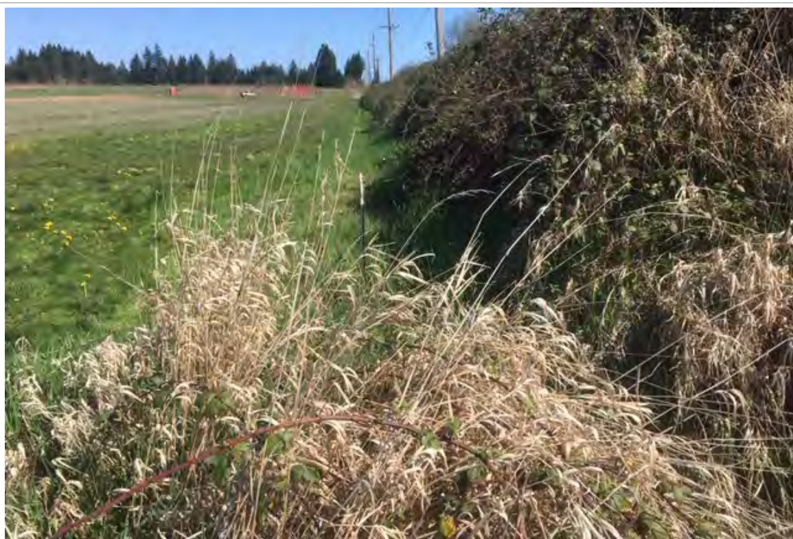
Photopoint 1: Below embankment along Dodge Park Boulevard. Steep slope down to agricultural field. Water collects along the slope and converges to this point, where water is collected in a culvert and exported.
