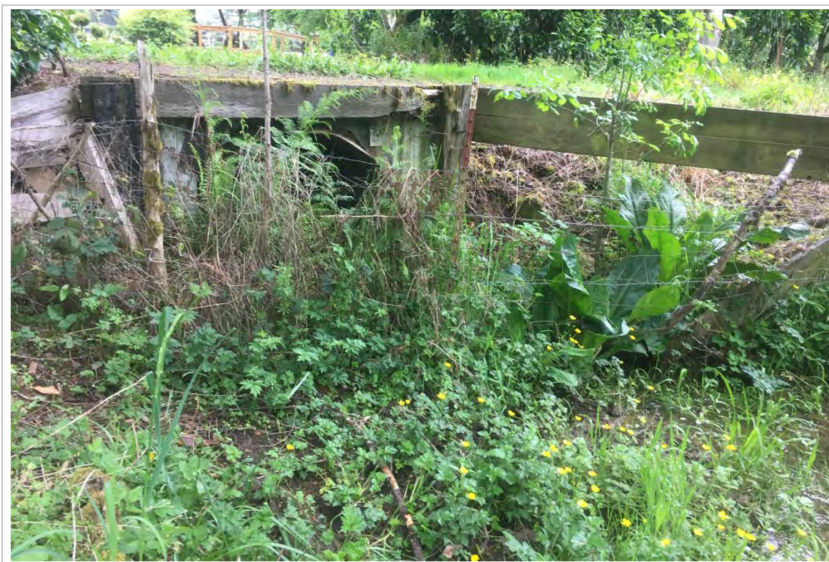
Photopoint 14: Driveway culvert at low end of drainage.
