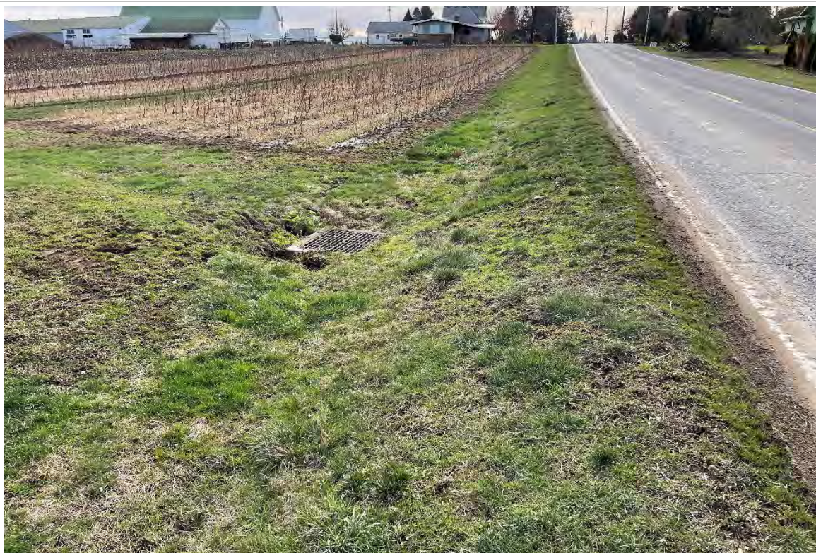
Photopoint 17: Roadside ditch on east side of Altman Drive, looking south. Vegetation is consistent along ditch. Green aerial signature is a drive aisle lacking evidence of flowing water. Water is captured in ditch inlet and flows west into drainage system. Plot 17 taken at ditch inlet (Routine OFFSITE)
