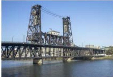
③ Steel Bridge
