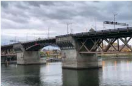
④ Burnside Bridge
