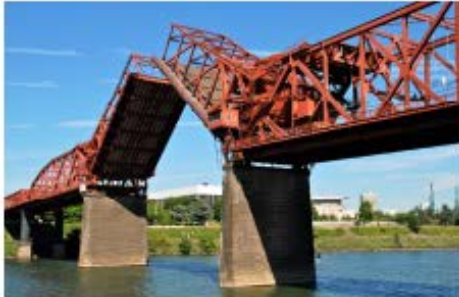
② Broadway Bridge
