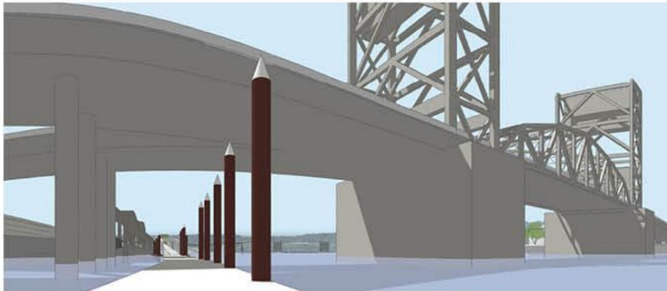
Long-span Alternative / Through truss / Lift
