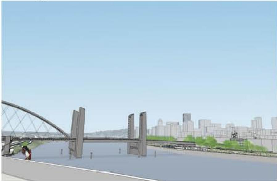
Refined Long-span Alternative / Girder / Cable-stayed / Lift
