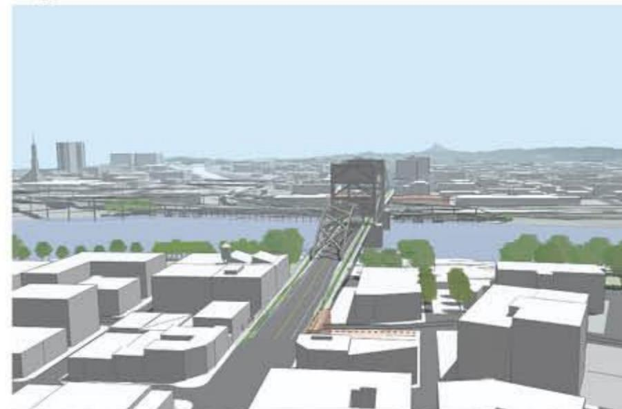
**Long-span Alternative / Cable-stayed / Lift**
