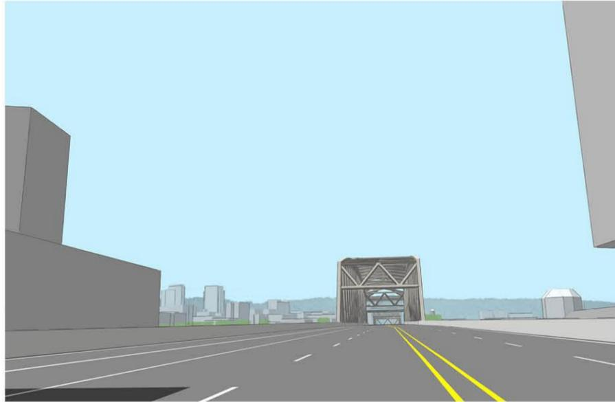
Long-span Alternative / Tied-arch / Bascule
