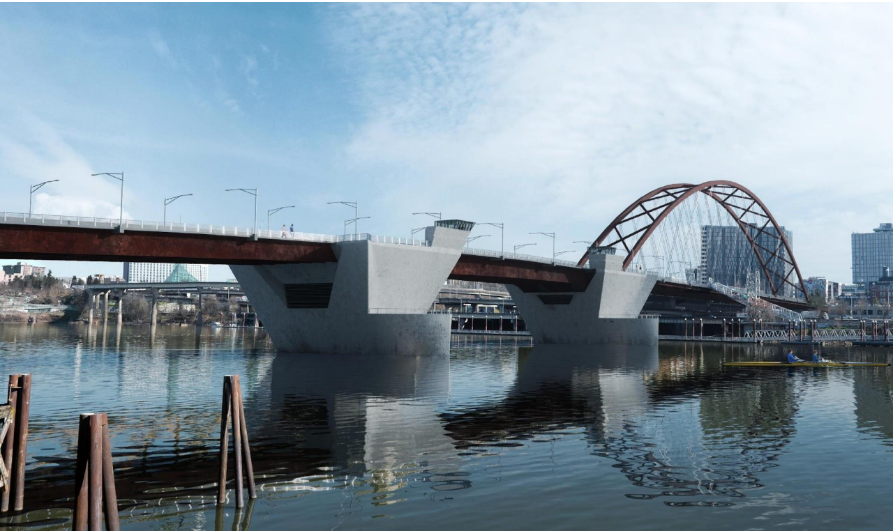
with Tied Arch for eastside long span
