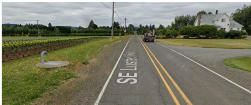
Figure 14. Example of Existing Air Vent and Access Vault (left) within Lusted Road ROW
